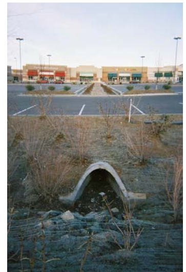
Alternative parking lot storm water management systems
