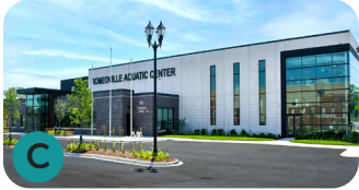
ROMEDEVILLE AQUATIC CENTER 630 TOWNHALL DRIVE
